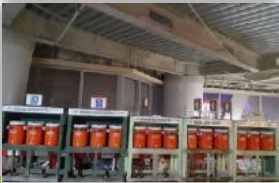
Drinking Water Station
